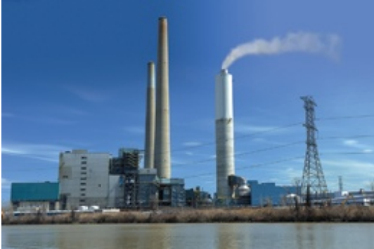
Coal fired Power plant with wet FGD, 7m stack on which extractive 181WS is installed
