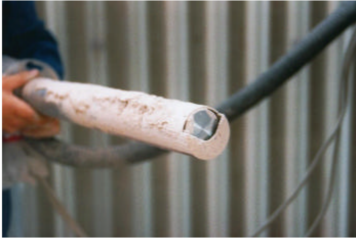
Fig 8 Use in raw cement gas
