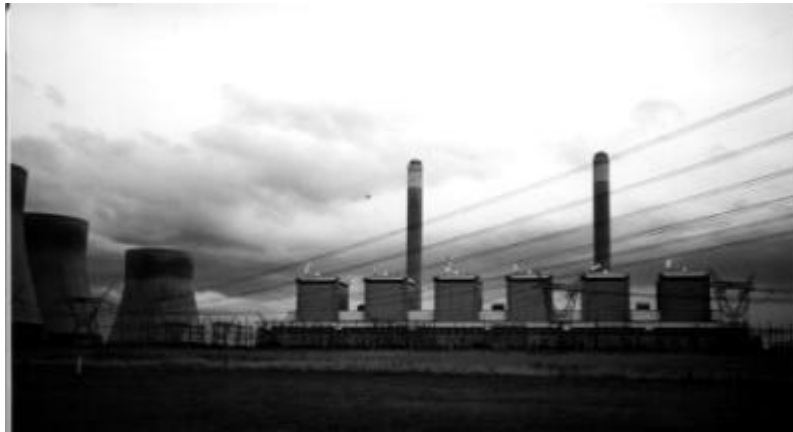
Figure 2. International Power Plant requiring “an approved” particulate monitor
