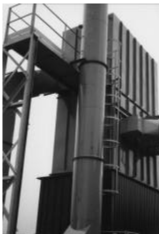
Figure 6. Typical small stack application on which small path length limits resolution of opacity instrument
