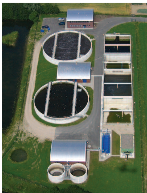
Figure 1: Aerial photo of the Glückstadt wastewater treatment plant
