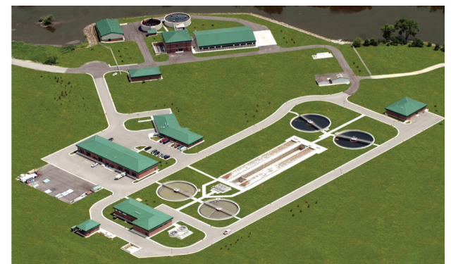
Aerial view of the Watertown WWTP
