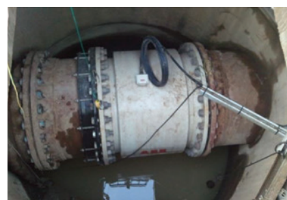
This particular flow meter a 900mm electromagnetic flow meter - one of the standard choices in the Water Industry
