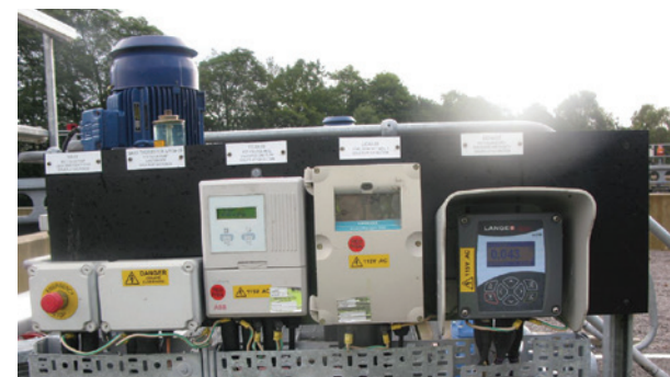
Just another choice of meters including flow, level & dissolved oxygen (left to right)
