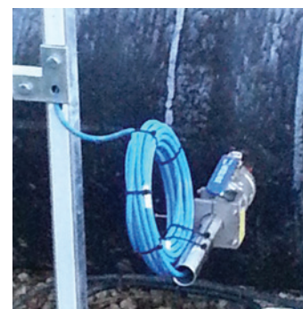
This particular flow meter a 900mm electromagnetic flow meter - one of the standard choices in the Water Industry
