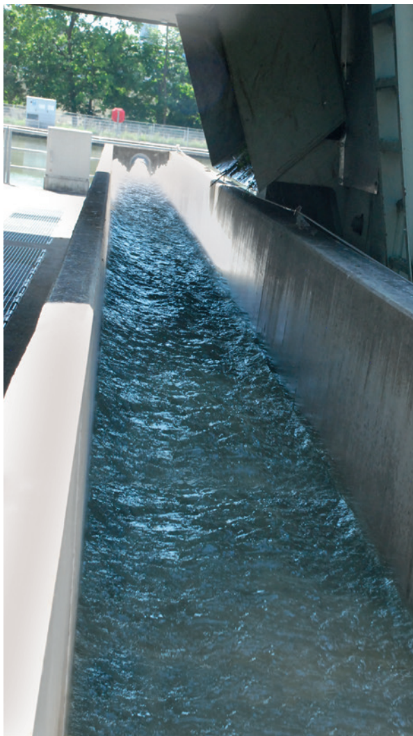
Like a big waste filter: the water that gets caught on the screen is returned to the Danube via a special channel.
