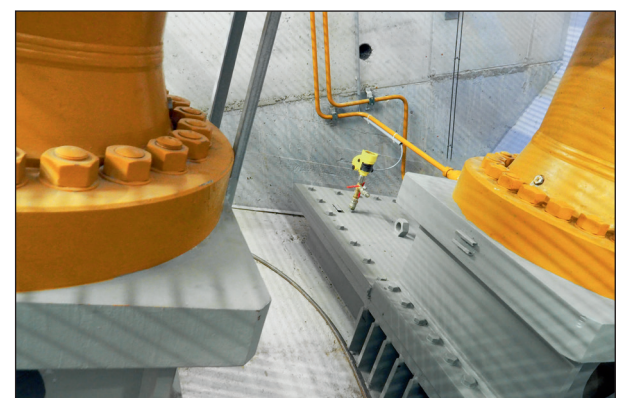
VEGABAR 82 takes on the task of redundant measurement, determining the water level in the reservoir with centimetre accuracy.
