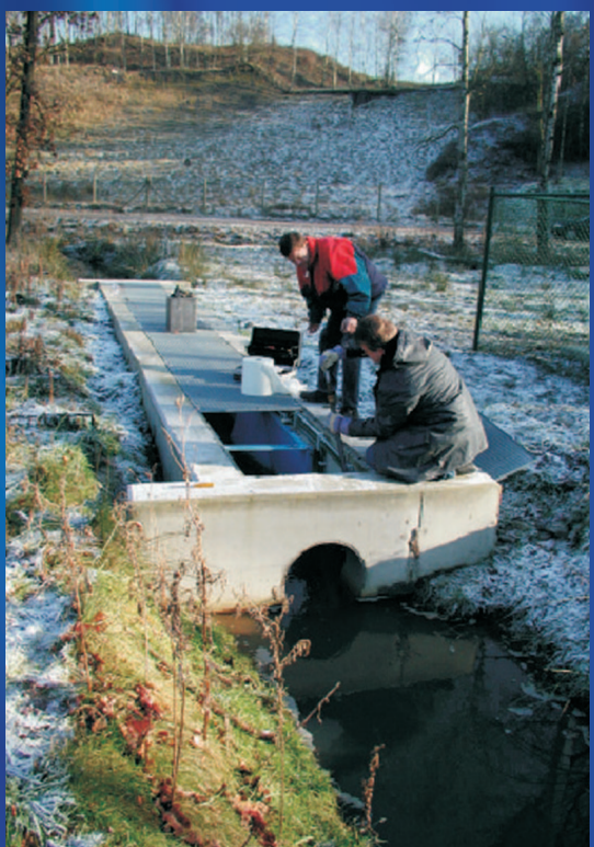
Fig.1: Carefully designed monitoring location with custom built flume.
