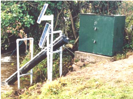
A WISER system installed in the field. The sensors are mounted inside and on the surface of the black plastic pipe. The data logger and automatic water sampler is inside the green cabinet.
