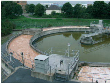
Fig. 1: Oxidation ditch with central final settlement tank
