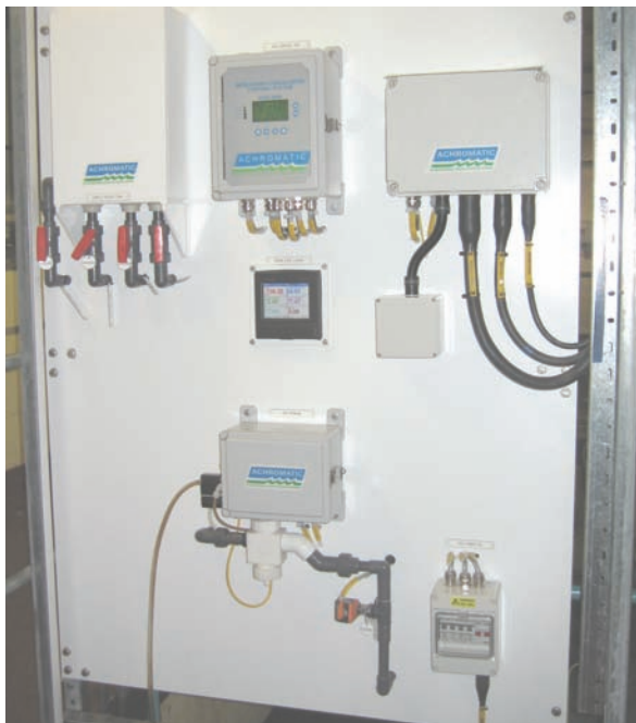
Figure 2b – ICCS 2000 Fully On-line Automatic Coagulation System
