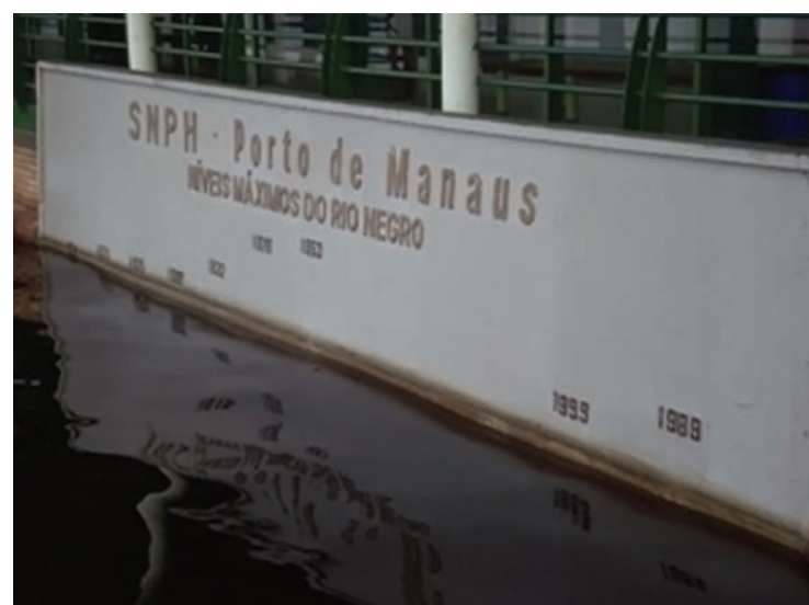
Figure 5: A wall on the Port of Manaus shows the highest flood marks of the Negro River. The Negro River and the Solimões River meet in Manaus to officially form the Amazon River. The highest mark when this photo was taken is from 1953. The 2009 flood surpassed it by about 15 cm (6 in) and peaked on July 5th. Photo courtesy of CPRM (Brazilian Geological Survey).
