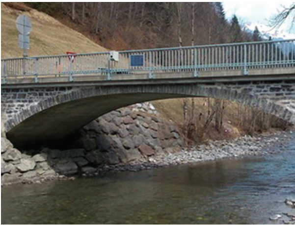
All-in-one RQ-30 station in the Austrian Alps. This unit can be operated stationary or mobile, for example during weather events with fast moving storm fronts. It contains an RQ-30, a data logger with mobile data transmission and an autonomous power supply in one housing. It can run on battery with an optional solar panel for longer monitoring periods. The unit may be deployed for a couple of days before it is moved to another monitoring site.
