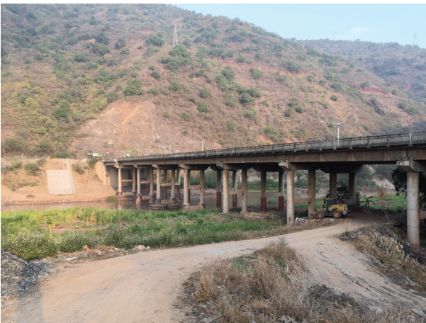
Application of a multi-sensor RQ-30d in China. Five RQ devices mounted to street lamps cover the whole river cross-section. One primary unit operates with five secondary units.
