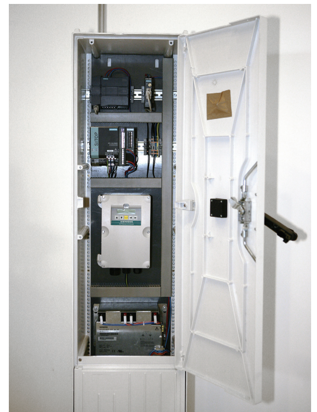
Figure 1: Siwa LeakControl system from Siemens including Sitrans FST020 transmitter for clamp-on flow measurement
