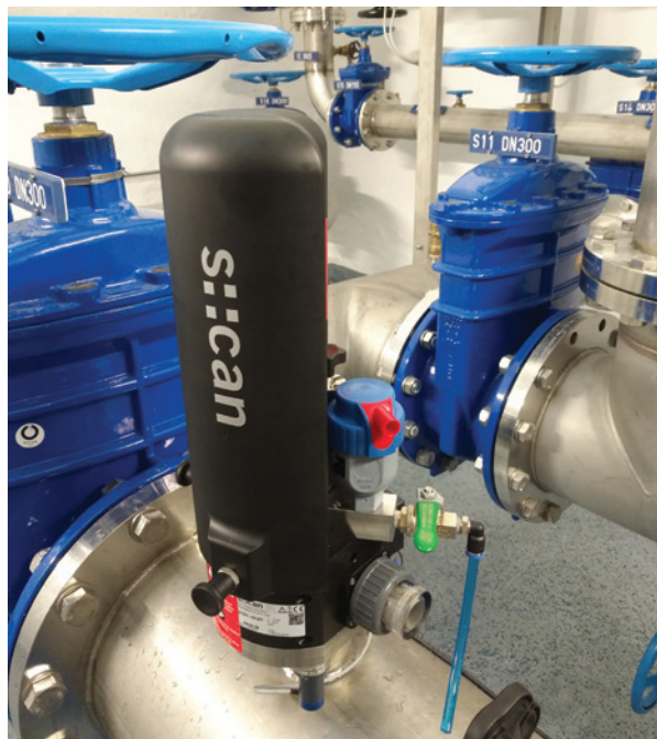
Figure 3: The cover of the pipe::scan provides additional security for the sensors and the operators
