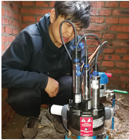
pipe::scan installation in a suburb of Beijing
