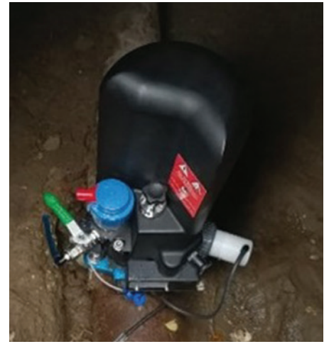
The pipe::scan is a sensor system for monitoring drinking water quality in pipes under pressure
