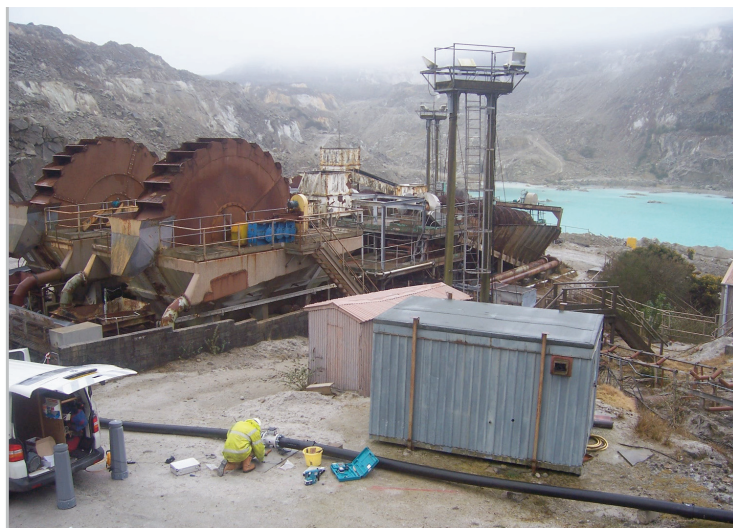
Installation of Flow Meter and Telemetry Outstation
