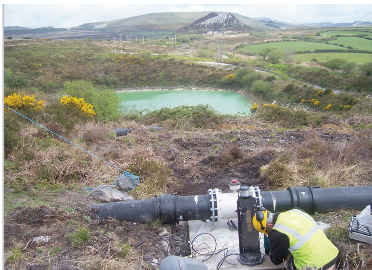
Fitting a Siemens Magflo Electromagnetic Flowmeter.
