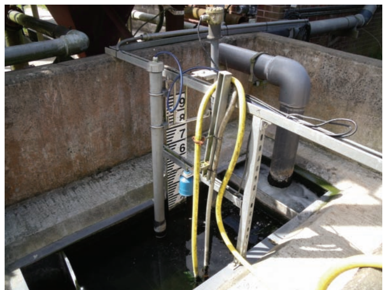
Figure 3: Where the flows from both aeration tanks merge prior to discharge, another Turbi-Tech LS turbidity monitor takes a final reading to ensure that the discharge consent level is not exceeded
