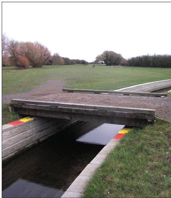
New channel increases hydraulic capacity. Image courtesy of MWH
