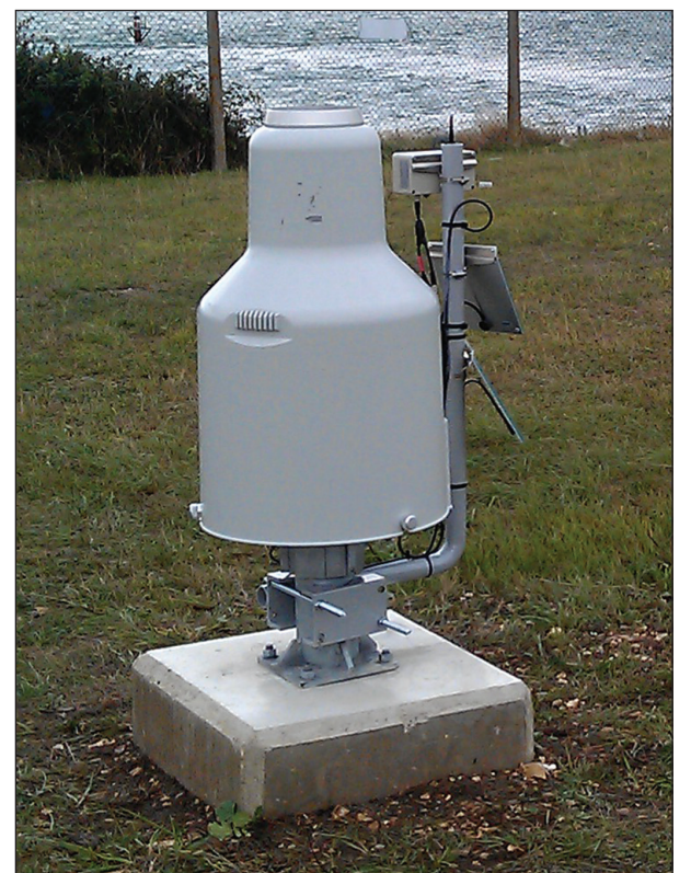
Solar Powered Pluvio 2 Raingauge with Adcon Telemetry
