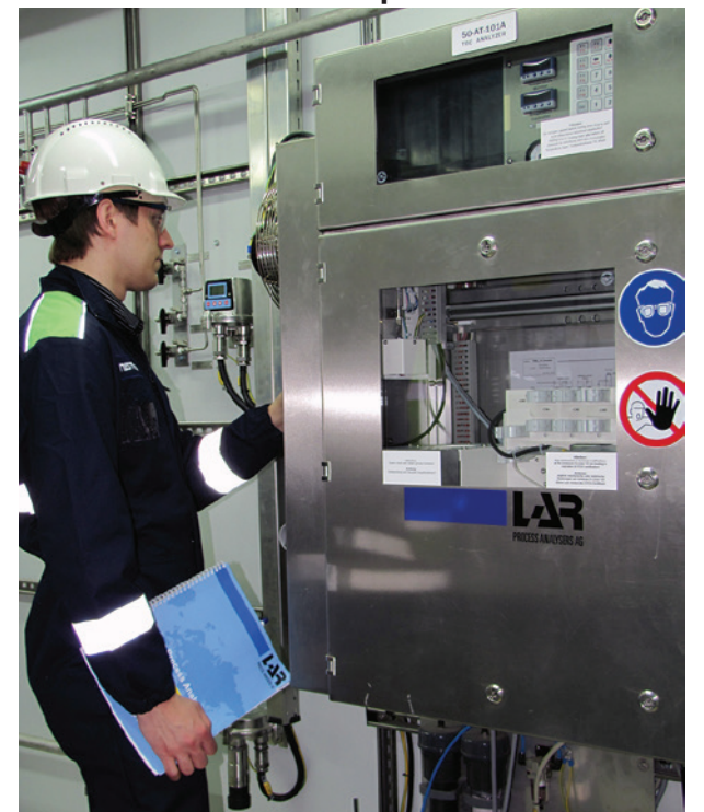
Inspection of a TOC-analyser in ATEX zone 1
