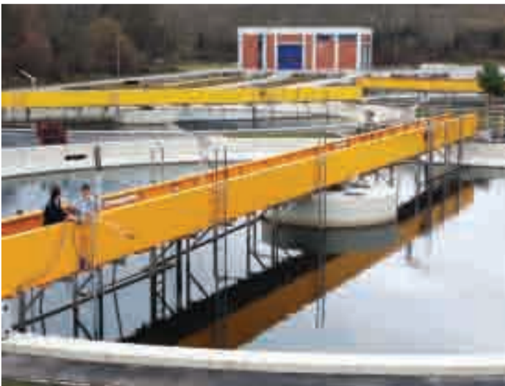
Final sedimentation basin of a municipal wastewater treatment plant today.
