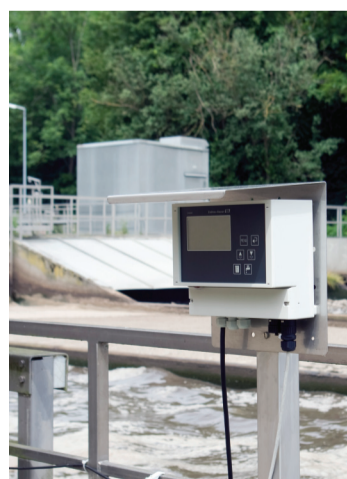
ISEmax used in the activated sludge basin of a municipal waste water treatment plant.
