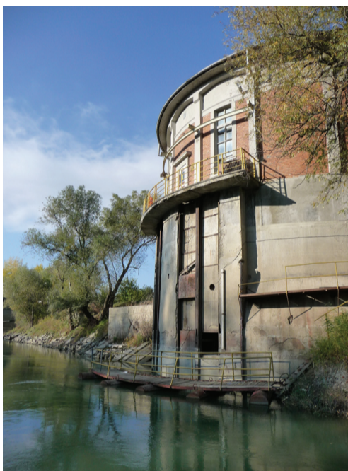
Figure 1: Water intake station on the Prut River.
