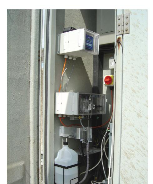
Measurement and control of  $H_2S$  levels after pre-treatment is vital because the presence of even low levels of  $H_2S$  will have a detrimental impact on subsequent biological treatment processes. Measurement at the discharge point is important to ensure compliance with legal requirements. PCB manufacture
