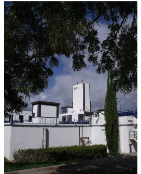
Fig 1 The Tavira water treatment plant and pumping station.
