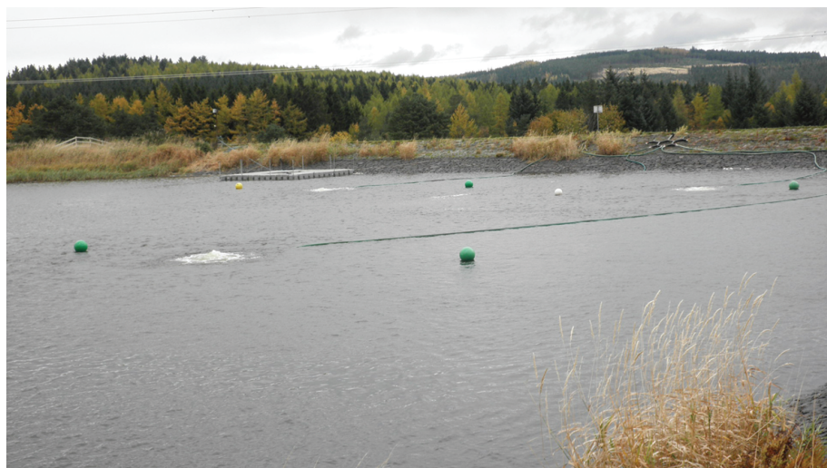
Craigshead Reservoir with Aquaerators in Action
