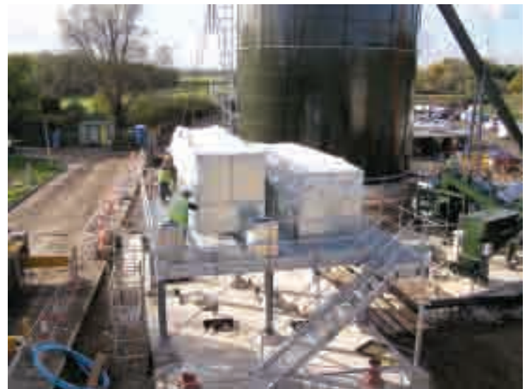
Outdoor installation of weatherproofed acoustic enclosure on centrifuge platform
