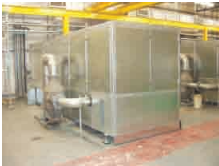
Indoor installation of acoustic enclosure around centrifuge
