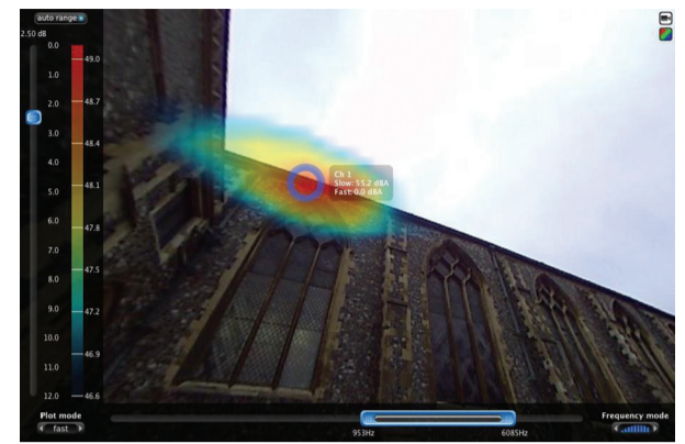
Figure 8: Acoustic leak pinpointed
