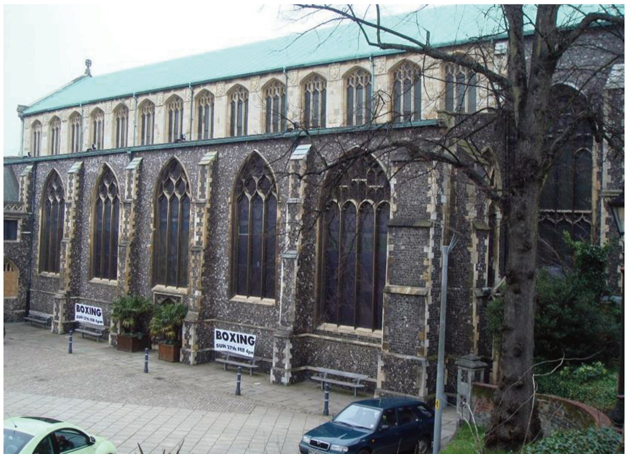
Figure 1: St Andrews Hall
