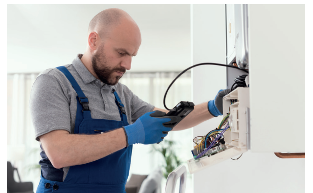
Testing flue gases from a domestic boiler
