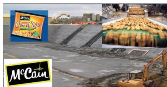
McCain Foods anaerobic lagoon in construction
