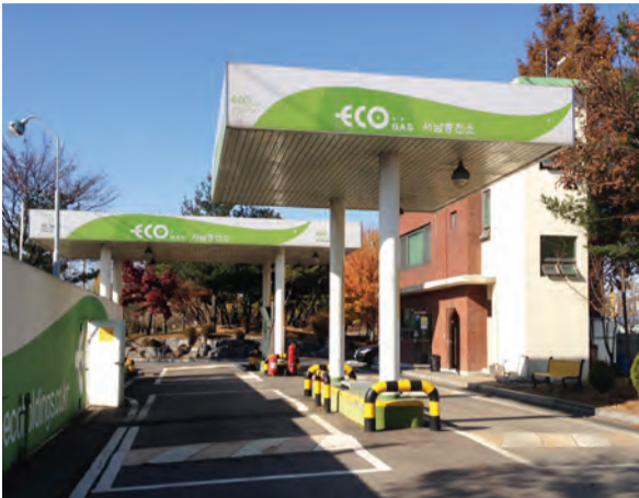
Eco Energy's CNG station in Korea
