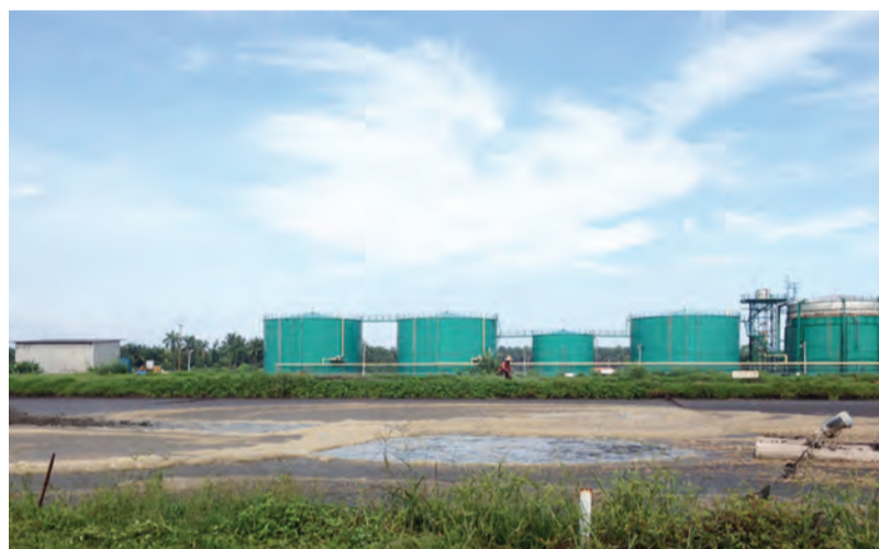
Palm oil waste water lagoon & digesters in Malaysia
