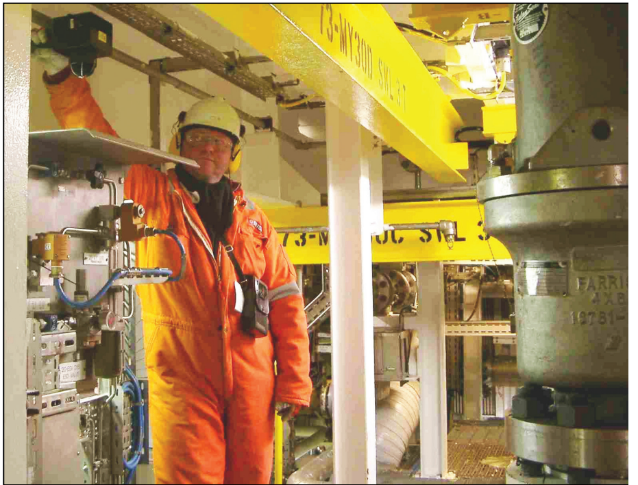
Figure 6: Innova Gassonic service engineer measuring the background noise
