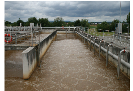
Figure 2. Waste water treatment plant
