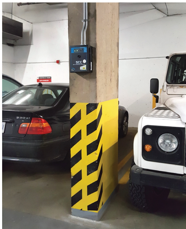
SCC-Car Park Installation
