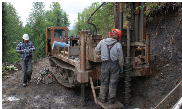
Figure 4: Drilling a monitoring well at Red Devil. (Photo credit Keith Torrance)
