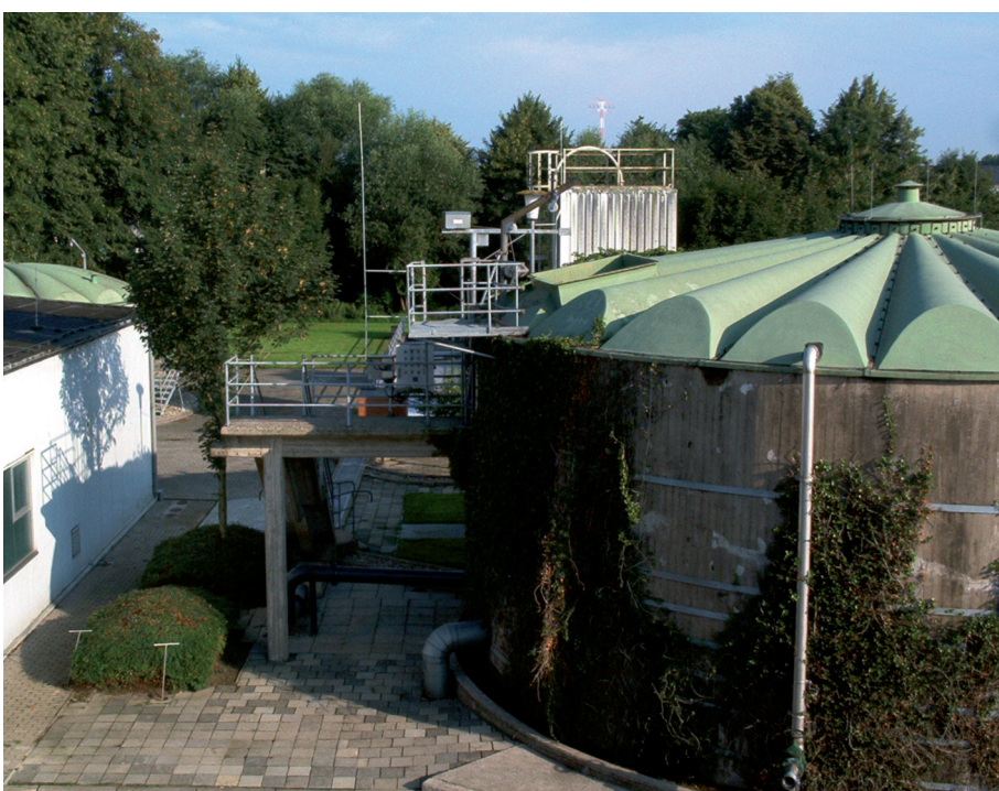
Fig. 1: WWTP Papenburg, Germany
