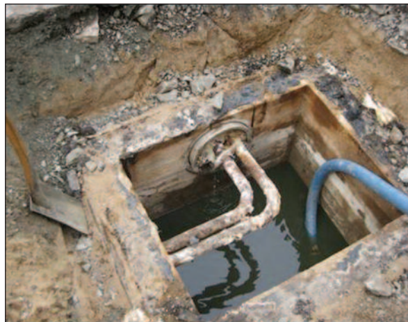
After seeing this leak in the report, the district heating company went there to investigate. It turned out to be a very large leak. Needless to say the company was very glad that this major leak was detected.
