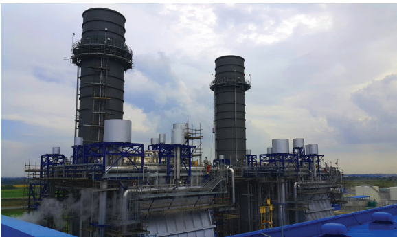
Gas turbine electrical power generation plant
