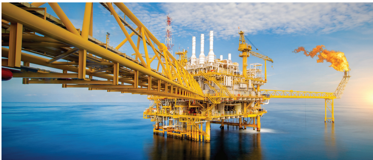
Gas production platform offshore
