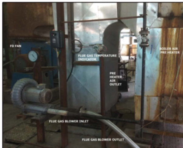
Figure 5. Effective use of Boiler flue gas for carbonation of process liquor at Tummalapalle Mill.
