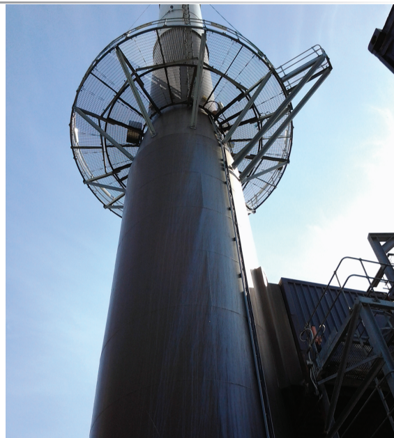
The stack and its gantry at the 30m level
