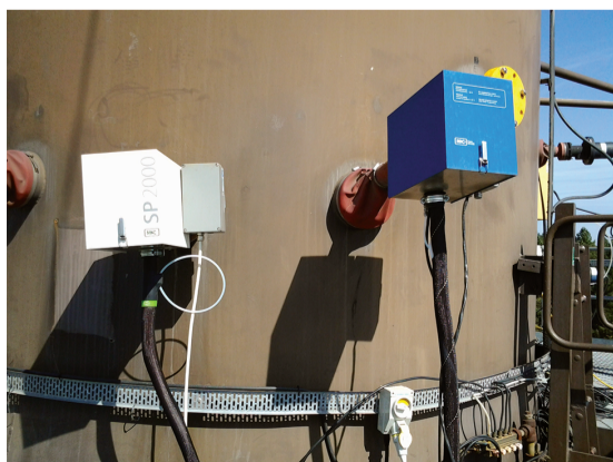
The prime AMS sample extraction probe on the right and the extraction probe for a 'hot spare' AMS system on the left
