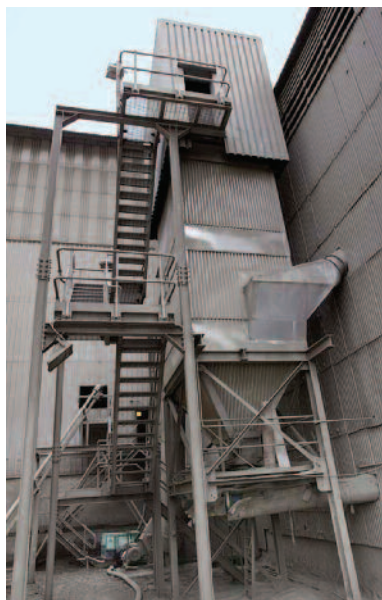
Cement Mill 45,000 m 3 /hr (25,000 CFM) 1.2m Stack
