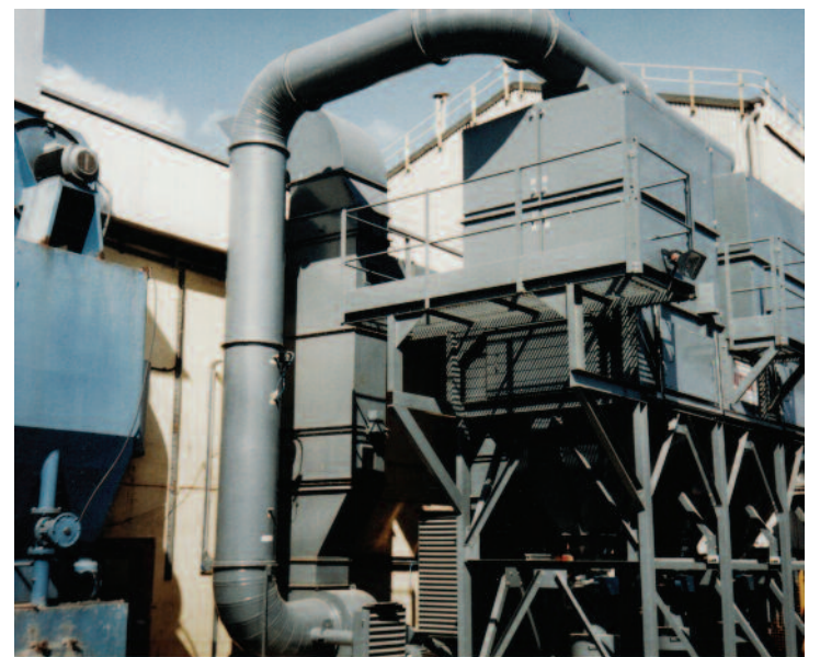
Battery Industry 27,000 m 3 /hr (15,000 CFM) 800mm Stack
