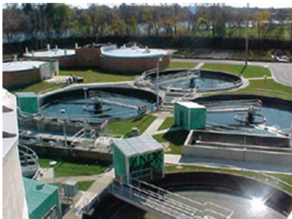
Industrial air monitoring waste water plant
